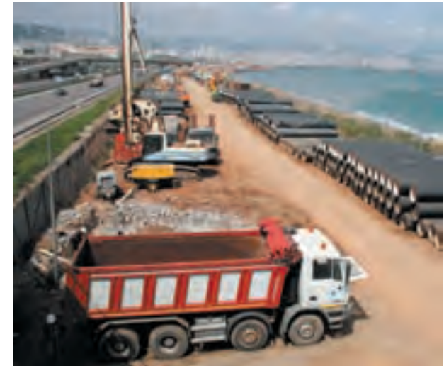
Building site of the Hamma desalination plant, in Algiers.
