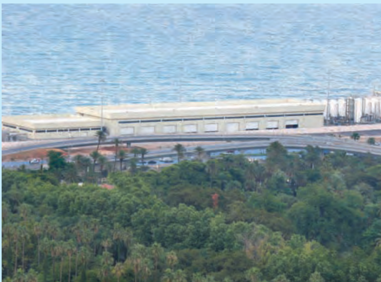
The station of desalination of Hamma (Algiers), inaugurated in January, 2008.
