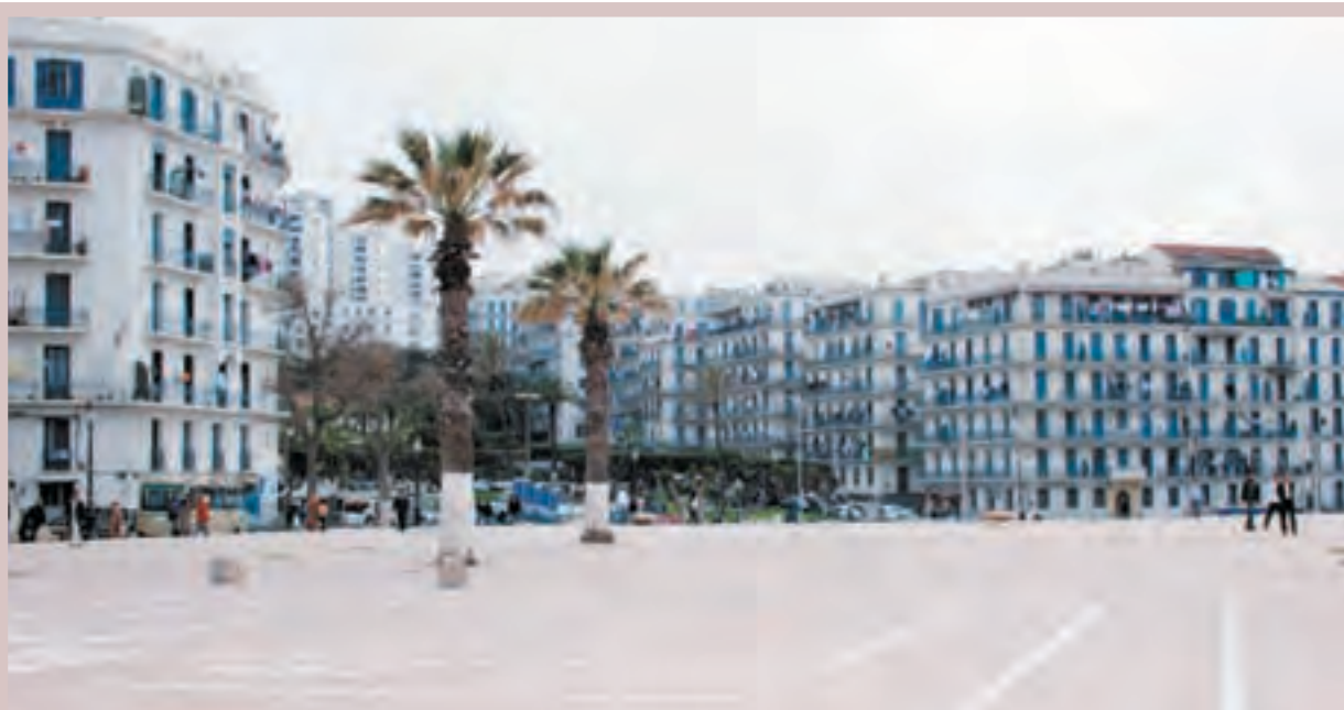
The new face of Bab El Oued.
