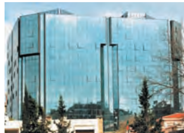
Sonatrach's headquarters in Algiers.
