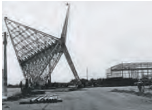
During the construction of the Palais des Expositions.
