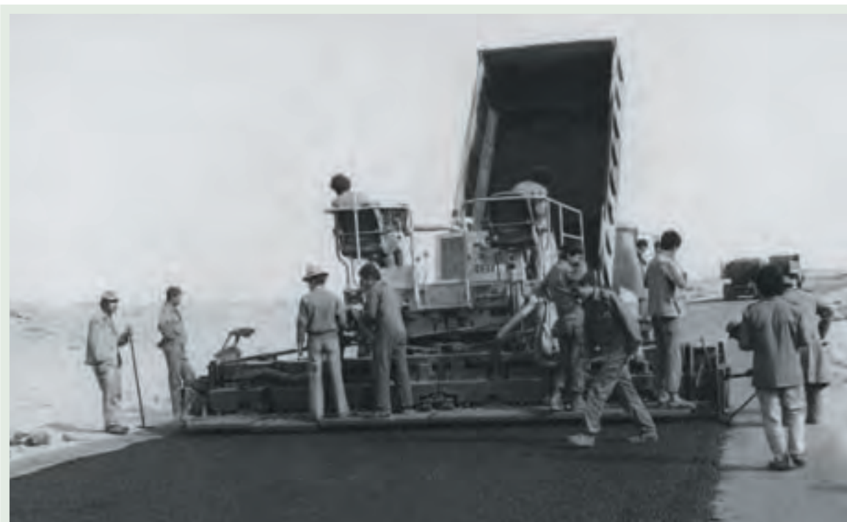
Asphalting operation of the trans-Saharan.
